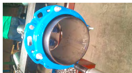
Tightening on the pipe.
